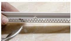
For an inside 90° miter, snip a "V" notch into the tear off strip.
