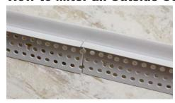
For an outside 90° miter, snip the mud leg all the way through the mud bump and the tear off strip. Do not snip the gasket.
