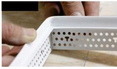
Make sure the front of the gasket is not snipped and bend the bead to ensure it forms a nice clean inside corner.
