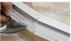
Next, flip the bead over and snip the mud leg all the way though the mud bump and into the back of the gasket.
