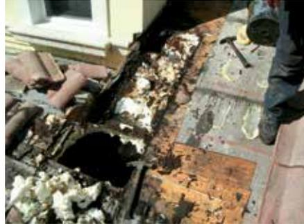
➤ OSB and plywood manufacturers, as well as the Engineered Wood Association, are beginning to provide recommendations to avoid the use of SPF under roof decks due to rot. (Photo credit: The Florida Roofing, Sheet Metal, and Air Conditioning Contractors Association)
