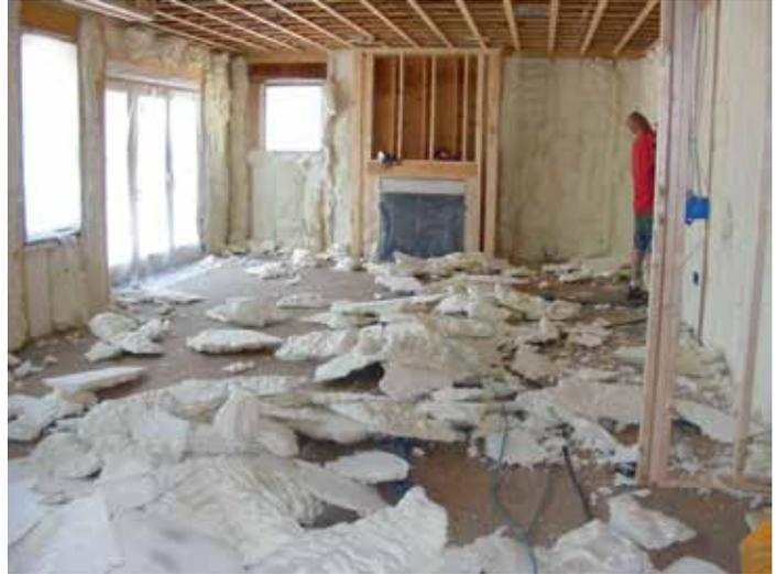
➤ Approximately one-fifth of the material used in a typical open cell SPF job is waste that goes to a landfill.<sup>2</sup>
