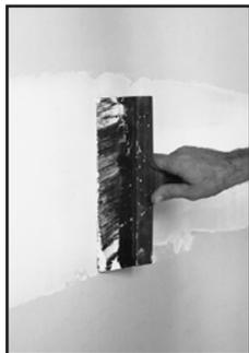
**Finishing coat.** Scrape, sand or use a damp sponge to gently remove any imperfections. Draw a 10" knife blade along the surface to ensure it is level. Apply a thin finishing coat to each joint, then feather outward 3" to 4" to eliminate imperfections.
