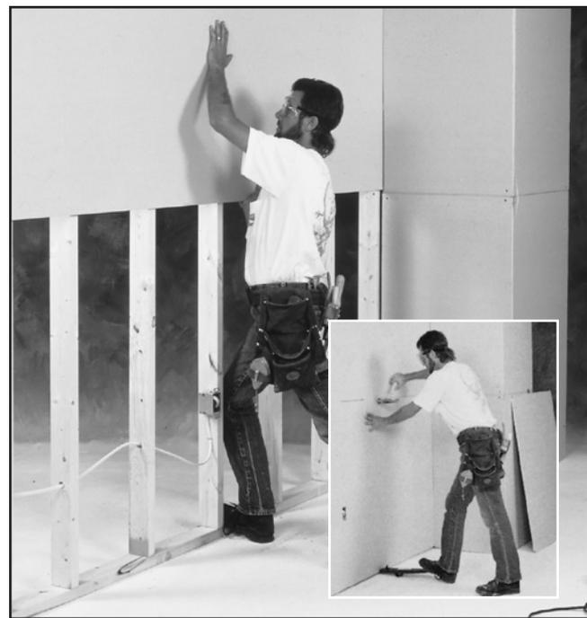
**Glue.** Even strong construction-grade panel adhesives must be reinforced with nails and screws. Make sure the framing surfaces are clean and free of contamination. Apply adhesive, following the manufacturer's instructions. Then use nails or screws, spacing them 16" apart in the field of the boards.
