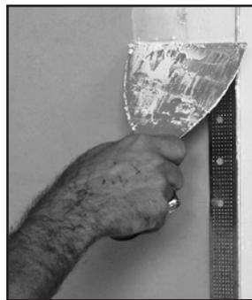
**Outside corners.** Using a 6" knife, apply the first coat of joint compound along one flange of the corner bead and smooth the compound outward with the knife. Repeat the process on the other flange. Allow the compound to dry and repeat the process again, using a 10" knife, feathering the edges outward.
