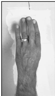
Dried pieces of compound will leave unsightly scratches, so throw away any compound that has dried pieces. While the compound is still wet, embed the reinforcing tape by centering the tape directly over the joint. Then use a 4" or 6" finishing knife to press the tape into the joint compound. Remove excess compound over and around the tape to level the surface. Let it set and dry about 24 hours.
