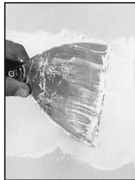
**Larger breaks.** Where the tape will not bridge the opening, use a key-hole or other saw to cut out an area around the hole. Cut the board back to the center of the stud on either side of the damaged area.
