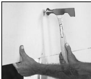
To install drywall horizontally (at right angle to the framing), start with the top board. Place together the tapered factory edge, moderately touching. Push the board firmly against the ceiling and fasten with nails or screws placed 7" from the interior ceiling angle. Space all nails 7" apart and screws 12" apart.
