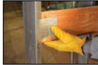
SNAP the Starter Edge into the open side of the flange
