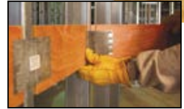
FLEX around stud flange using the flexible connector plate
