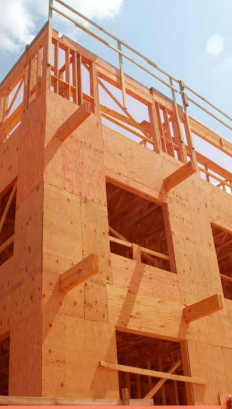
Since 1981, Dricon<sup>®</sup> fire retardant treated (FRT) wood has performed as intended in countless structures around the world, providing a convenient and economical building alternative. Pressure-treated for protection in the event of a fire, Dricon<sup>®</sup> FRT wood reduces flame spread and smoke development, the #1 killer in fires.
