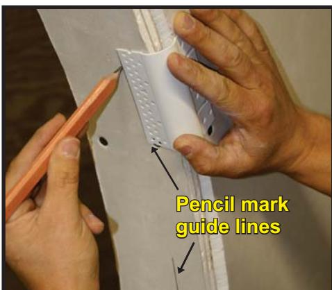
Begin by cutting a short piece of the Bullnose No-Notch Arch as shown to the left. Use this piece to draw guide lines along the length of the arch. The guide lines are used to ensure a straight installation. Make sure the legs are properly aligned and not splaying out as shown to the right.
