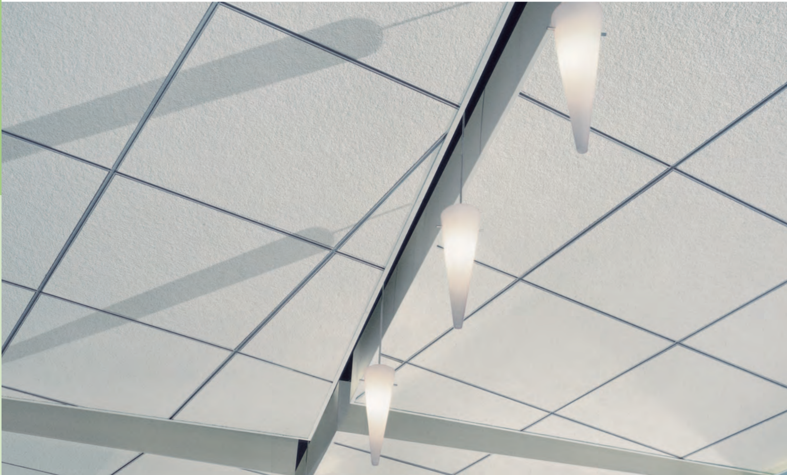
Eclipse Panels with CLIMAPLUS Superior Performance/ DONN FINELINE DXF Suspension System
