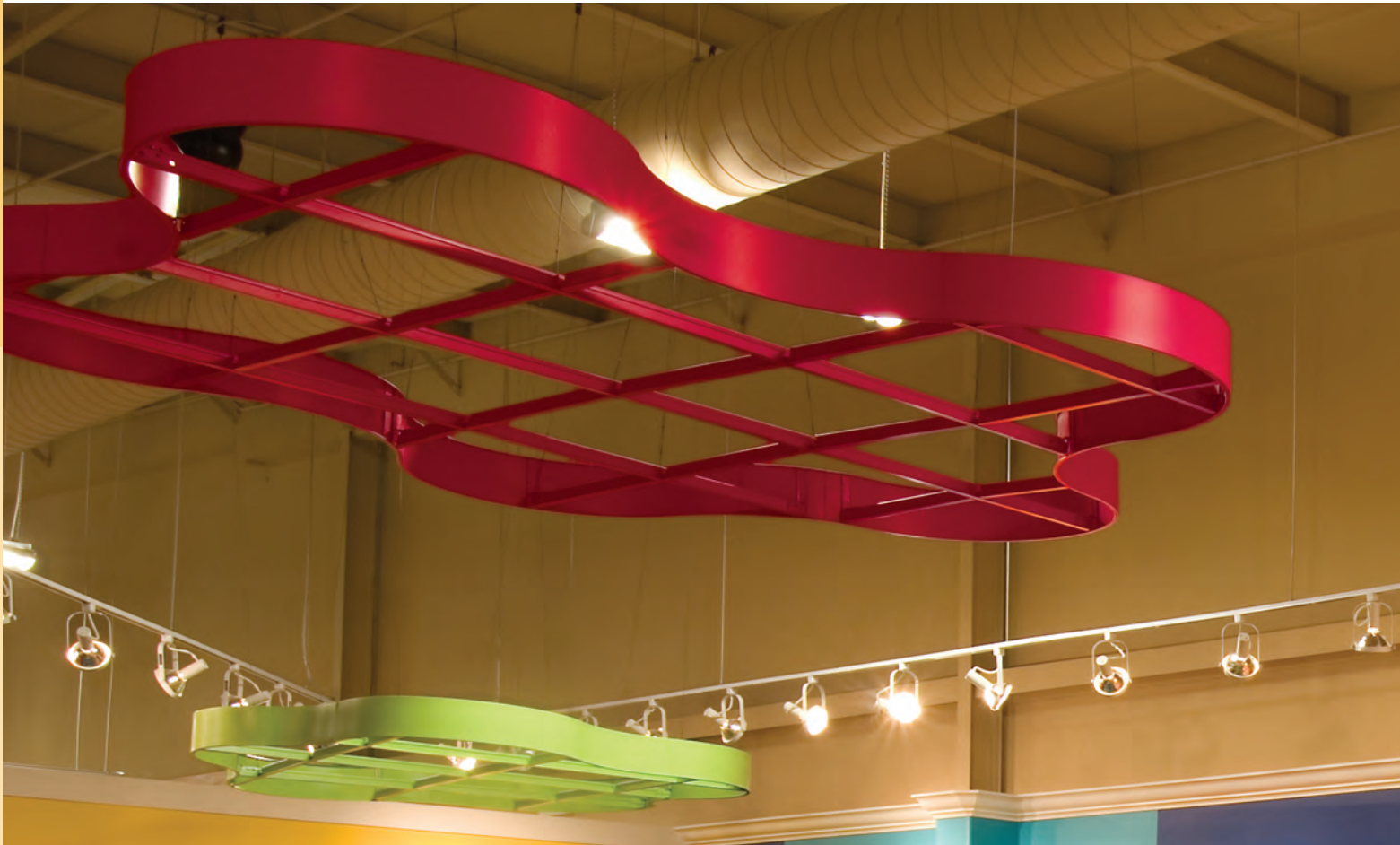
GRIDWARE Suspension System (GWDXW) with 2' x 2' Cells in Custom Colour/ 8" COMPASSO Perimeter Trim in Matching Colour
