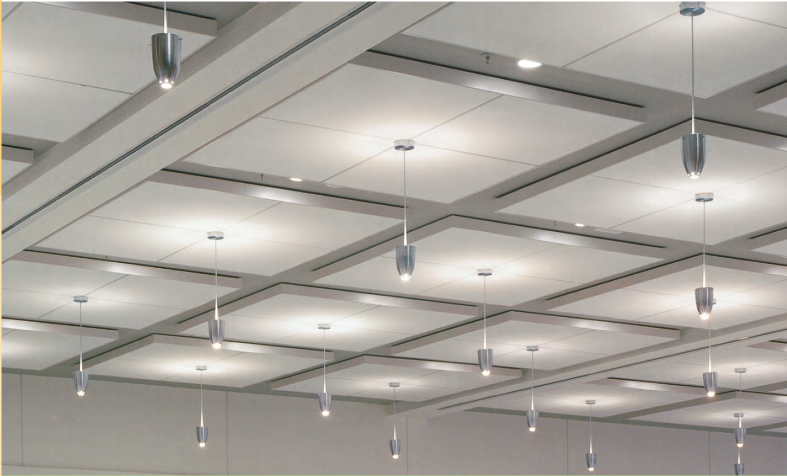
COMPASSO Perimeter Trim with HALCYON CLIMAPLUS Ceiling Panels/ DONN FINELINE DXF Suspension System
